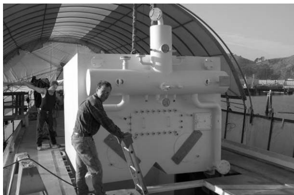
Figure 8 - New Rentech boiler being lowered into the engine room by Steve Cobb.
